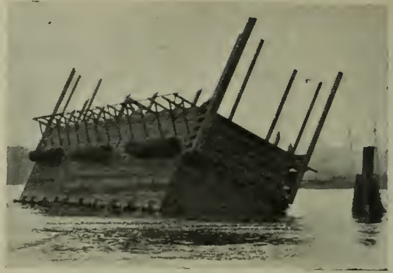
FIG. 4. COUNTERWEIGHT TRUNNION PIER CAISSON SINKING INTO POSITION.
